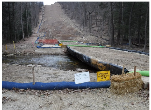
Pipeline Construction at Laurel Run, Perry County. Photo Courtesy: D. Weaver
